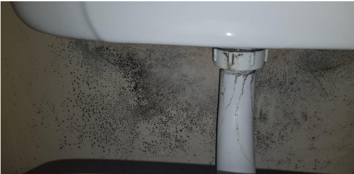
Figure 17: Mould in Flat 3 arising from persistent damp and condensation around cold water pipes in an uninsulated and unheated bathroom
