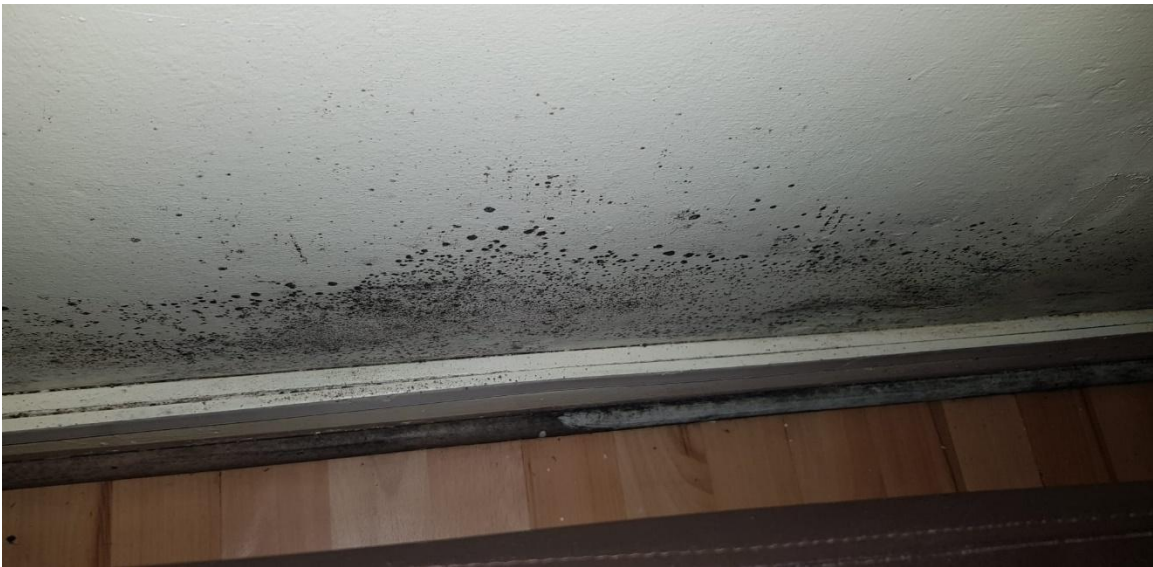
Figure 18: Mould in Flat 3 on cold and damp exterior walls
