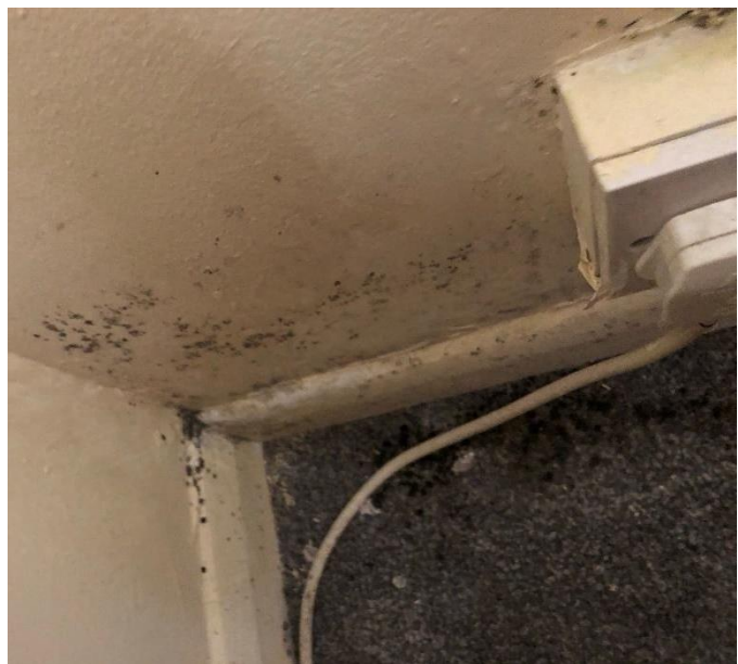
Figure 18: Mould in Flat 3 on cold and damp exterior walls
